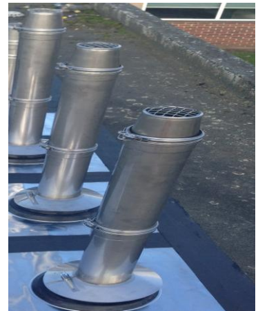
External View of flue termination
