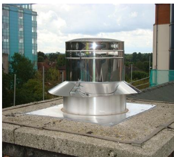
View of Chimney Top
