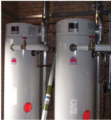
Internal Flue Systems
