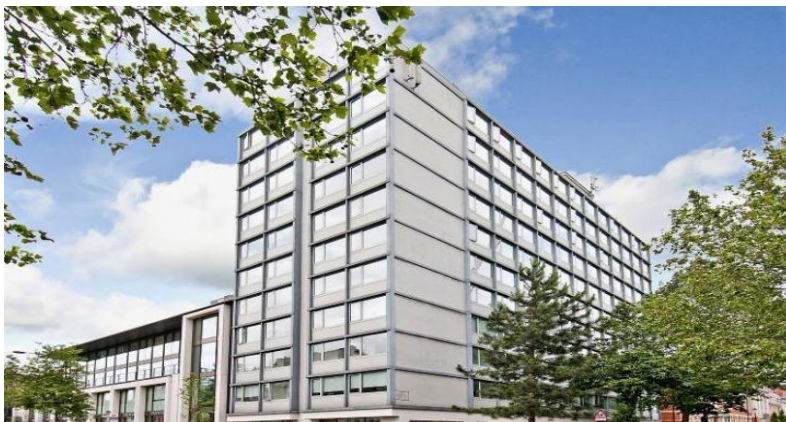
External View of Building
