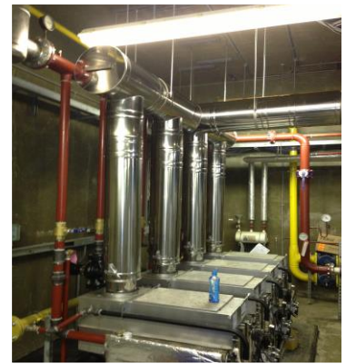
Installation of twin wall flues
