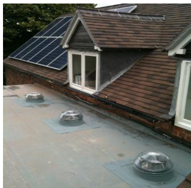
Solatube Systems (rooftop)
