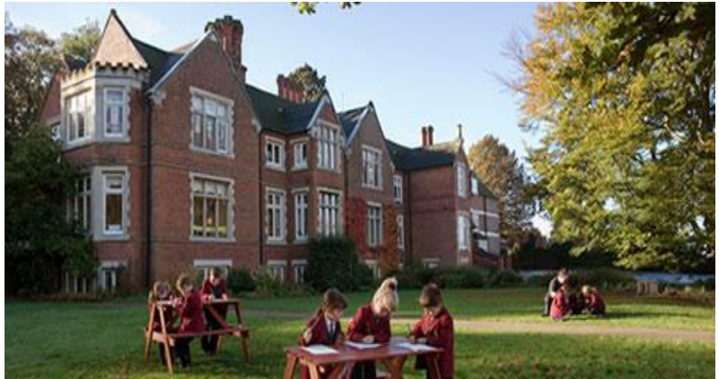
External View of Building
