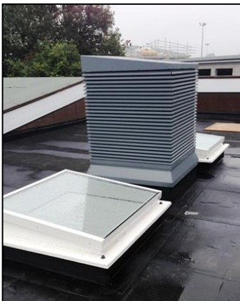
External view on flat roof
