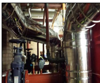
Internal Installation of flues
